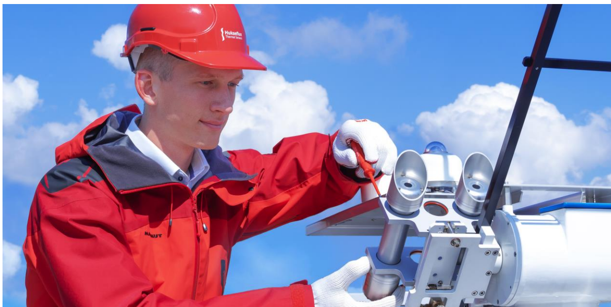
Figure 0.2 Application of DR20-A1 and DR15-A1 pyrheliometers, here with SR15-A1 pyranometers, in a typical solar radiation monitoring station
